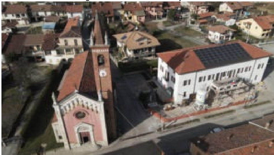
Figure 7 - PV installation on City Hall.
